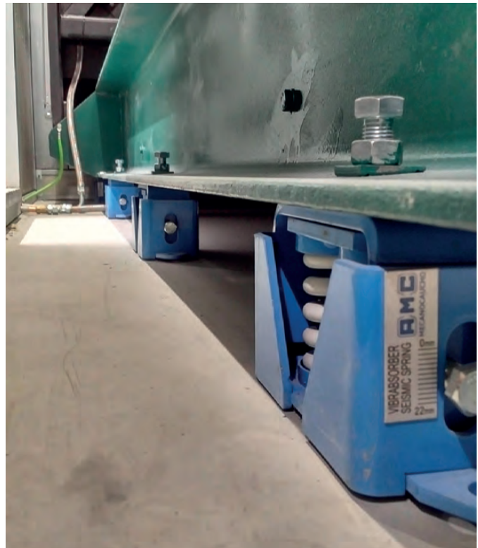
Compressor insulated with VIBRABSORBER +Sylomer®
