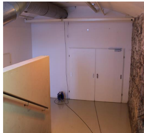
Picture 3: positioning of the acceleration sensor on the plasterwork of the brick arch
