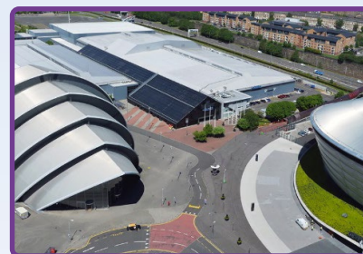
SEC Aerial View
